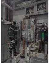
For installation in hazardous areas, the Control Panel is designed with Exd Ex-proof enclosure for a small heater load and/or Contactor controlled where heat dissipation is minimum. These are usually for local Control Panel use in tank immersion heaters.
