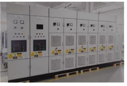
A Control Panel is installed to the Electric Process Heater to operate the heater throughout the lifespan of the system.
