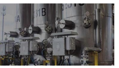
A Hot Water Calorifier is akin to the hot water heater at home. It is used for hot water supplies to the living quarters, mainly in offshore applications. Our advantage is being able to supply complete products with an in-built heater.
