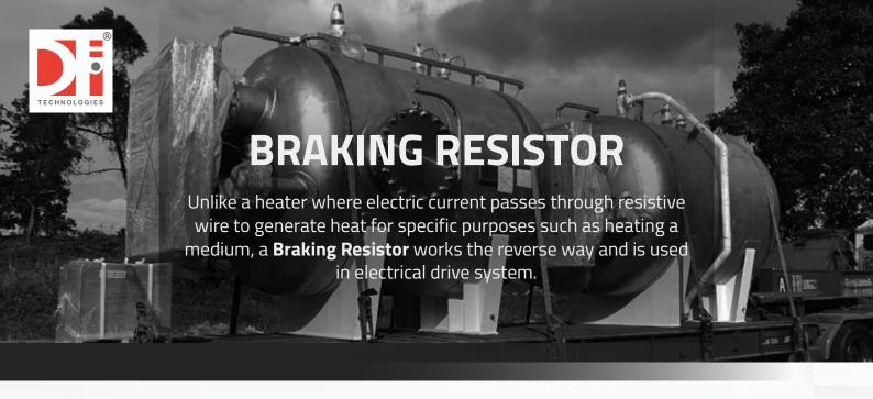
When a machinery is required to stop, the action of decelerating of the motion transforms kinetic energy into electrical energy and this process is known as dynamic braking which can be either **regenerative braking** or **rheostatic braking**.
